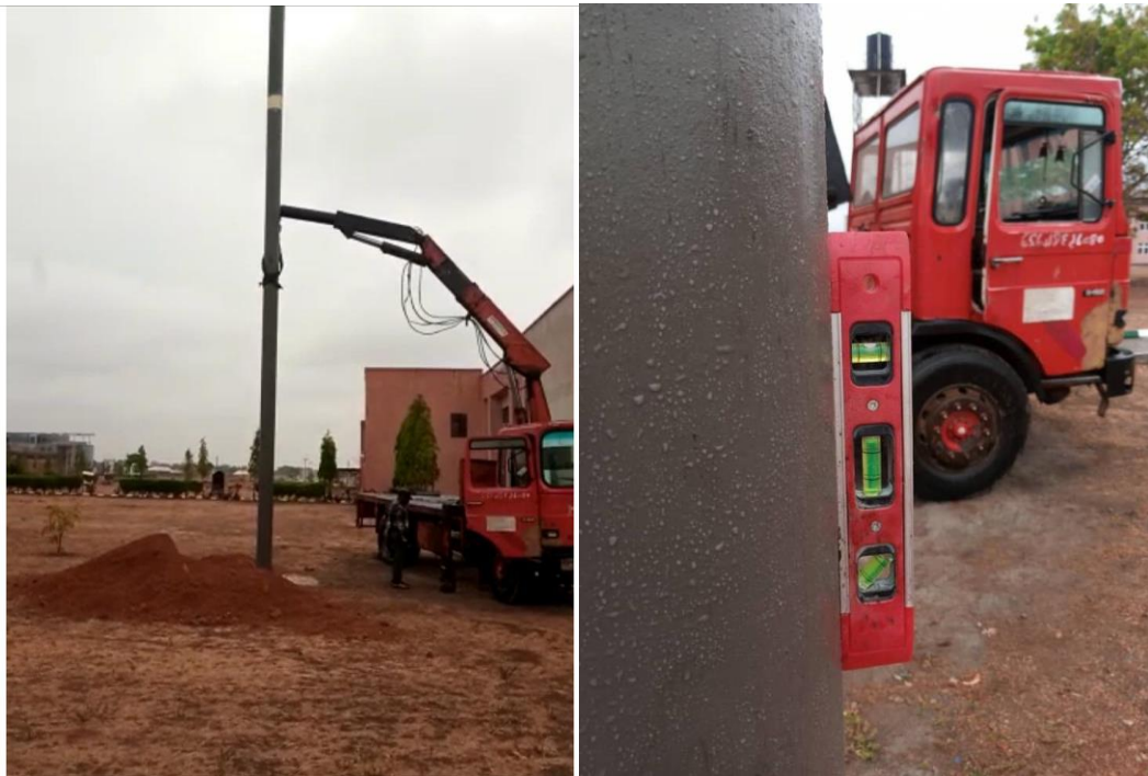
Plate 3.9b Alignment of the tree trunk
